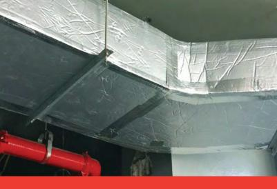
Closed cell, physically crosslinked polyolefin foam insulation with ultra tough foil facing to prevent mechanical damage in high risk areas.
